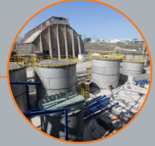
Stok Tank Storage Tank
